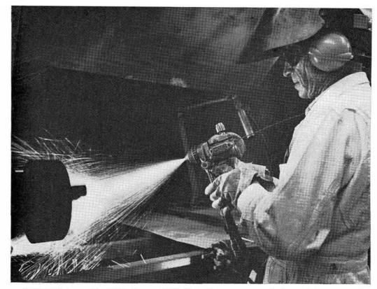
WIRE GUN is used by Fidel Chavez (4221-2) to flame spray a cylinder with high carbon steel. The process is equally suitable for applying thin coats or for resurfacing worn parts. Various combinations of ceramics and metals are possible.
